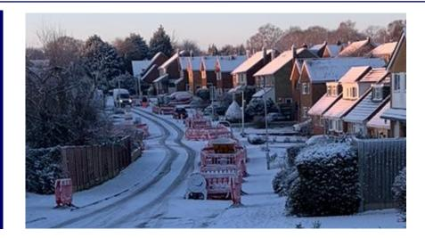
This scheme was caried out to rehabilitate existing water mains in the Draycote area of Rugby and involved the replacement of 10,224m of 75mm - 250mm dia Asbestos Cement, Cast Iron and UPC Water Mains in 23 separate roads under Severn Trent Water's AMP7 Lot 2 'Build Only' framework.
